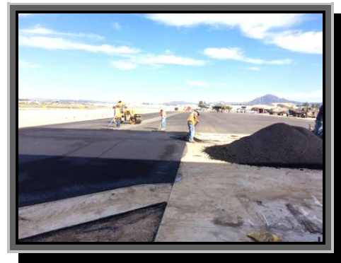
© Photo by Dan Newcomb Workers spreading the asphalt & rolling it.
