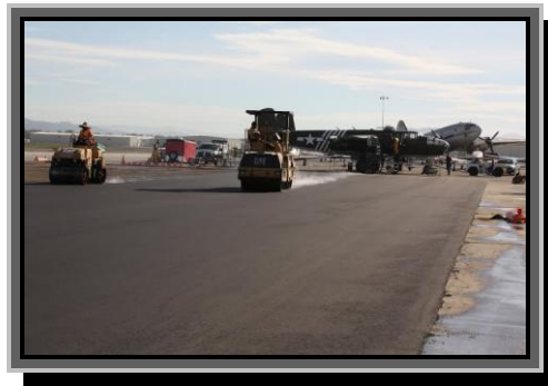
© Photo by Gene O'Neal The finishing rolling of the ramp to make it smooth
