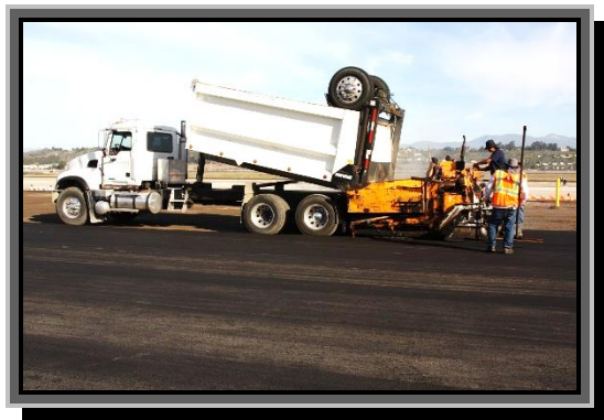
© Photo by Gene O'Neal Trucks dumping asphalt to be spread and rolled
