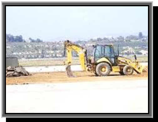
© Photo by Dave Flood Breaking up old ramp & levelling ground
