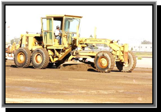
© Photo by Gene O'Neal Earth-moving machine leveling off ramp
